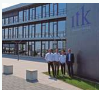
ITK Engineering GmbH. An innovative office building located in Germany. ECOi - PACi
