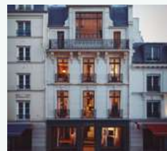
LIAIGRE showroom, well-known as a luxury design architect in Paris, France. ECOi
