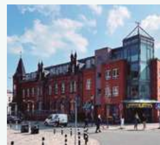
The EDEKA store in Germany, the first supermarket providing the maintenance-free nanoe™ X technology for better indoor air quality. Germany. ECOi and nanoe™ X
