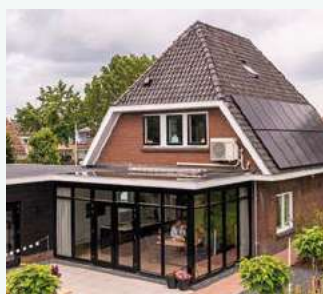
Aquarea T-CAP provides a complete solution of heating, cooling and DHW for the refurbishment of a luxury house in Voorthuizen, Netherlands. Aquarea
