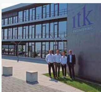
ITK Engineering GmbH. An innovative office building located in Germany. ECOi - PACi
