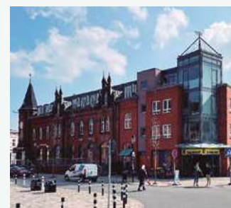
The EDEKA store in Germany, the first supermarket providing the maintenance-free nanoe™ X technology for better indoor air quality. Germany. ECOi and nanoe™ X
